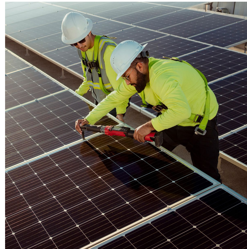
Technicians from Simmitri perform maintenance on solar panels installed at Bench-Tek Solutions in Santa Clara, California. Both companies are alumni of the Apple Impact Accelerator.
